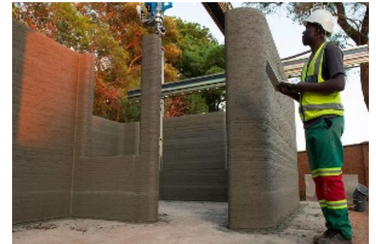
In Malawi and Kenya, companies like 14Trees have been able to build a 3D-printed house in just 12 hours for under $10,000. The reduced construction waste almost tenfold and reduced CO2 emissions by up to 70% relative to a standard house-building project. A 3D-printed school has also been completed.
